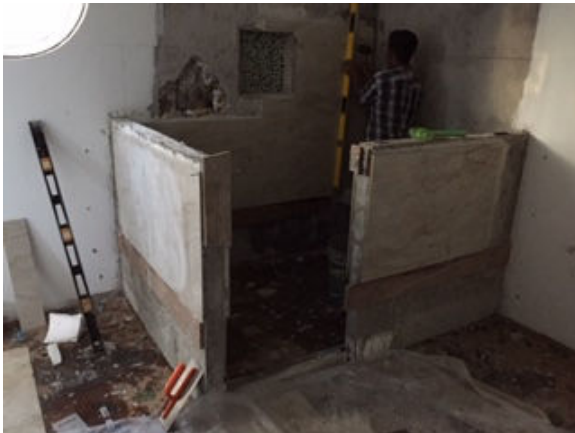
Installation of Floor and Wall Tiles to Bathrooms.
