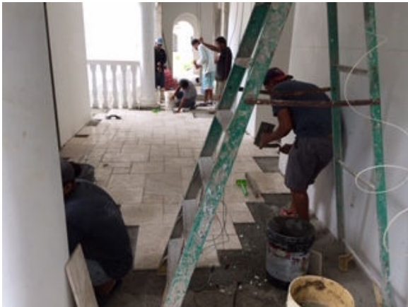
Installation of Floor Tiles and Base Tiles to Balconies.
