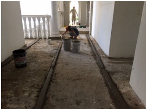
Installation of screed lines and filling up with concrete to allow for Tiling.
